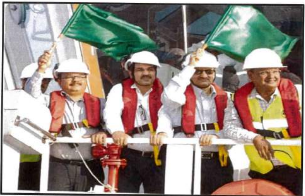
FIRST LOT OF STONES, PLACED AT SEA BOTTOM ON 28 TH JAN 2021 MARKING THE BEGINNING OF A JOURNEY TOWARDS COMPLETION OF BREAKWATER
